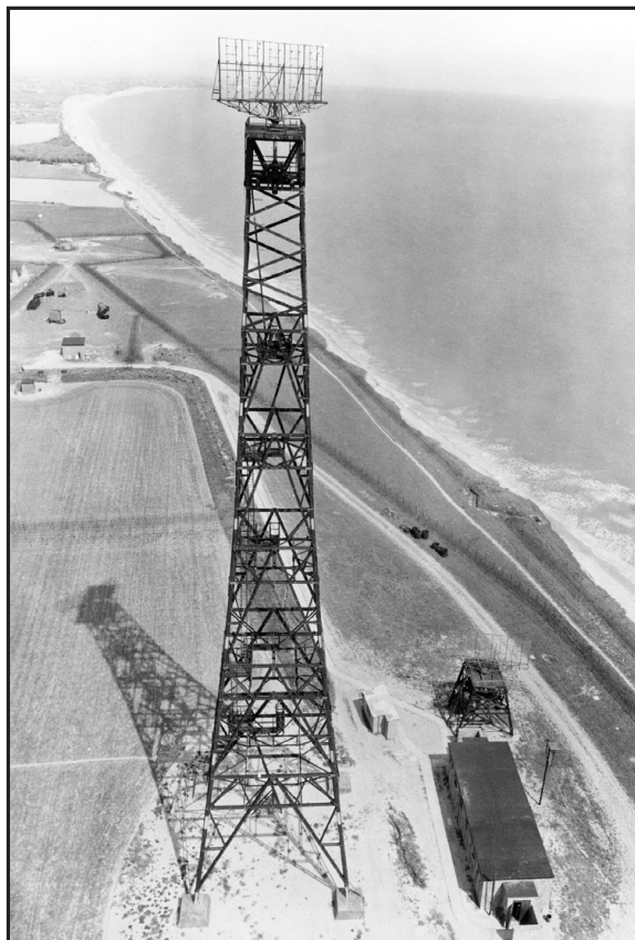
CHL radar installation at Hopton-on-Sea
